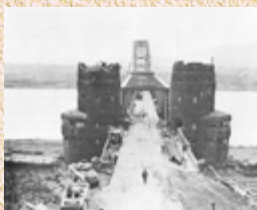
LUDENDORFF RAILROAD BRIDGE AT REMAGEN
