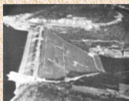
THE SCHWAMMENAUEL DAM
