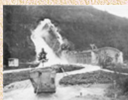
DAMAGE TO THE SCHWAMMENAUEL DAM causes flooding of the Roer River.
