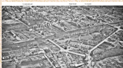
CROSSING SITES AT DUEREN
