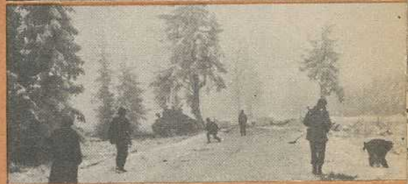
No one envied the job of the armored engineers. Above, that 540 foot trestleway across the Seine. Center: engineers pull the teeth of the Siegfried Line with TNT. Bottom: an icy road in the Ardennes is carefully searched for mines, one of which has already knocked out the Sherman in the background.
