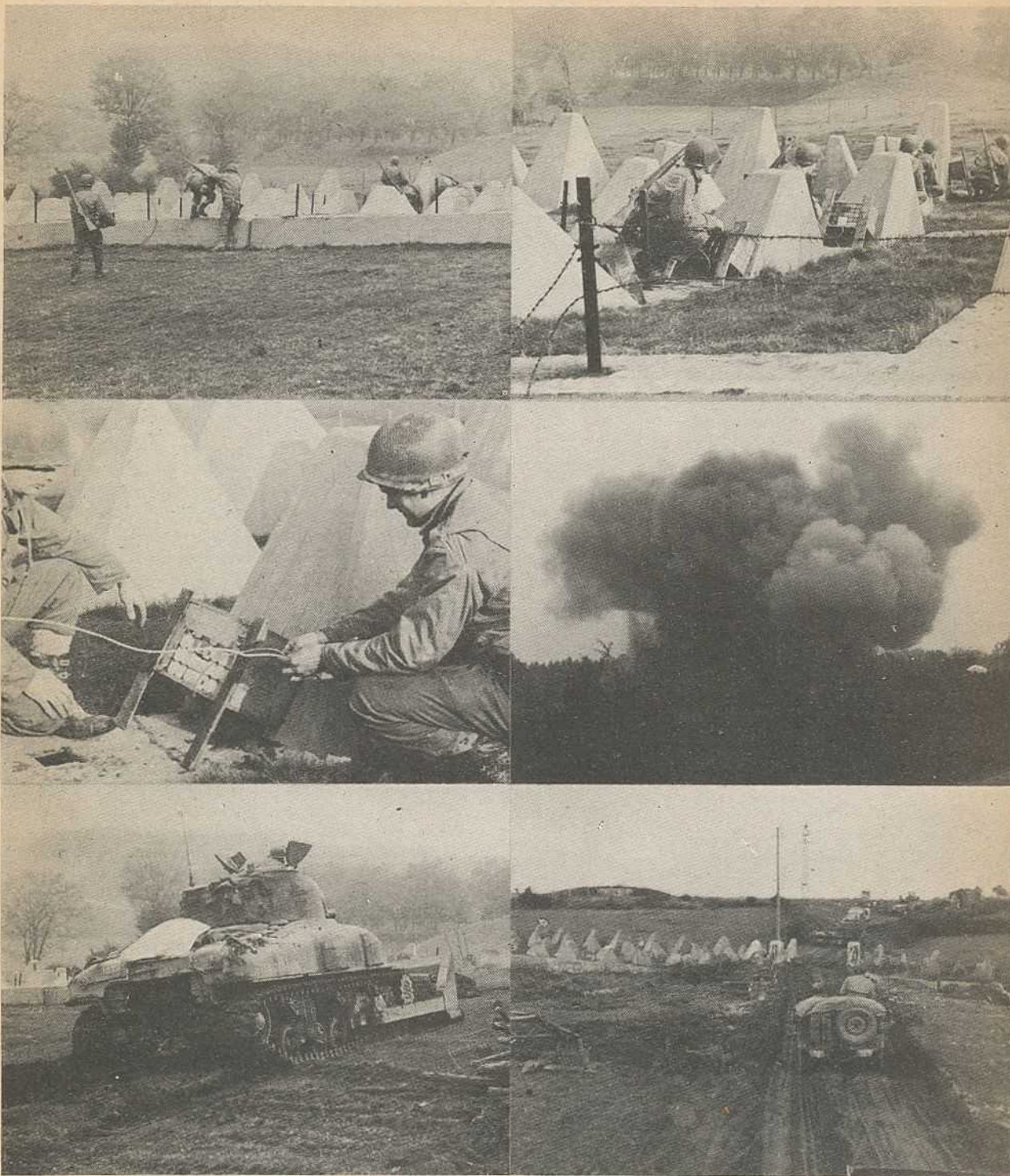
The men of "C" Company, 23rd Armored Engineer Battalion, demonstrate obstacle breaching technique on the Siegfried Line after the fighting has moved on into Germany. First the section moves forward to place TNT against the separate dragons teeth in the area to be blown. After demolition has been accomplished a tank-dozer smooths the way and - there you are: another hole in the famous west wall.
