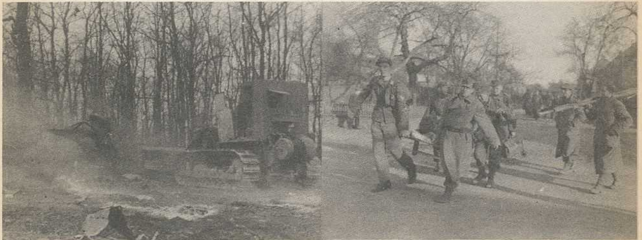
The roads were often blocked with wrecked and burning vehicles of the Wehrmacht. A bulldozer cleared the right of way.
